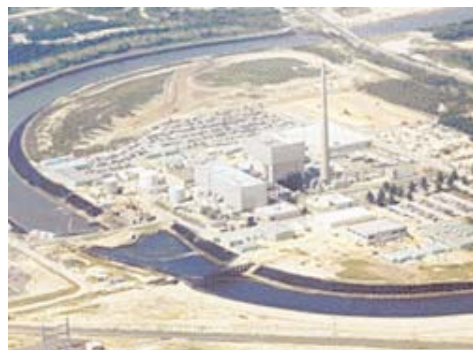
Oyster Creek Nuclear Power Plant
